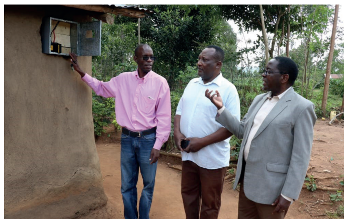
Kakamega County Supervisor Mr. Daniel Onyango and CECM for Roads, Public Works and Energy CPA Geoffrey Omulayi inspecting the completed REREC Projects
