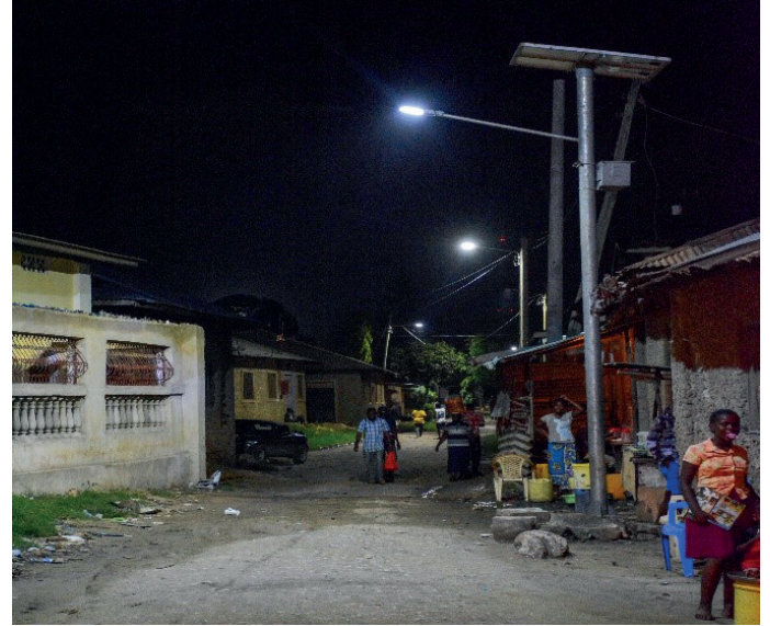
Some of the installed solar streetlights in Nyali Constituency.
